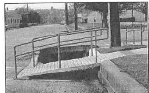
Plenty of street width is available for an imaginative solution to curb ramp installation at this small town intersection. Open culverts extend several feet from the curb at cross streets and are bridged with concrete ramps, open below for drainage, and handrails for edge protection. Beginning at the top of the curb almost 15 inches above road grade, these flying ramps both protect the culvert and provide access to the crosswalk. Edge protection is needed, however, and detectable warnings at the street edge.
