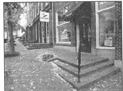
This streetscape improvement in a historic downtown works with the street slope to provide individual entrance platforms at existing businesses. Level landings on the upside connect back to the downside with steps. A clear passage of 1.5 m (5 feet) is maintained between the furniture zone at the curb and the stepped entrance platforms.
